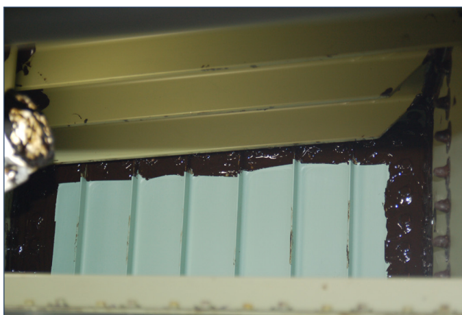
Door Installation and Sealant Coating
